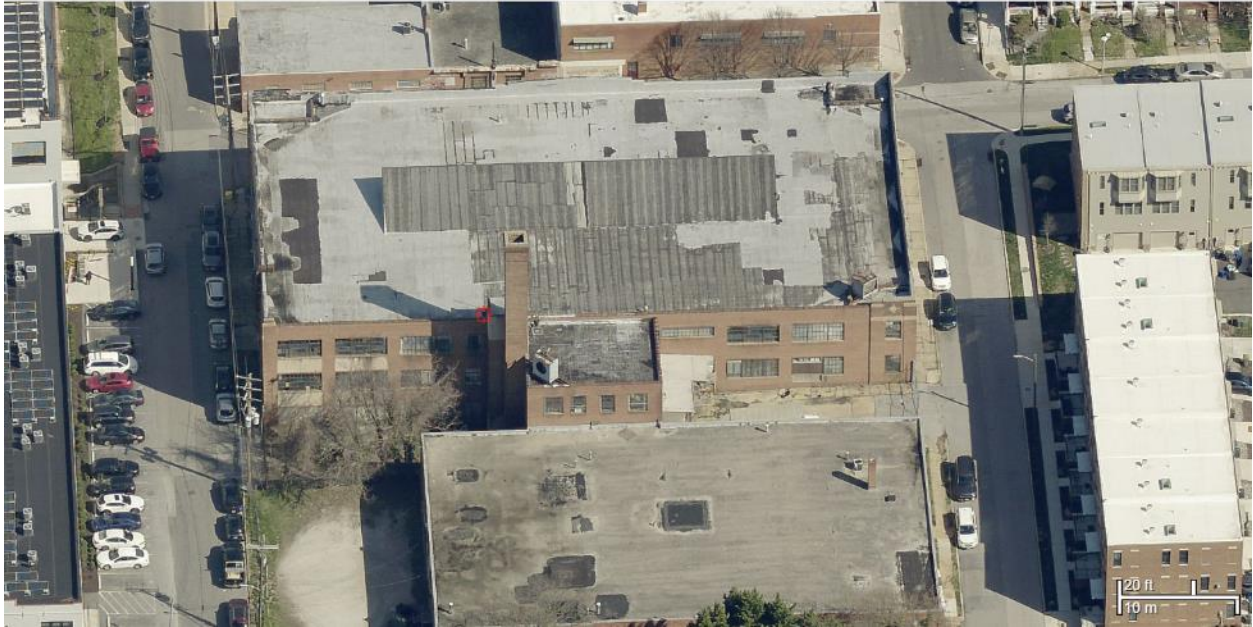
Image 7: Aerial view of 3110 Elm Avenue from the south, zoomed-in. Connect Explorer, April 2022
