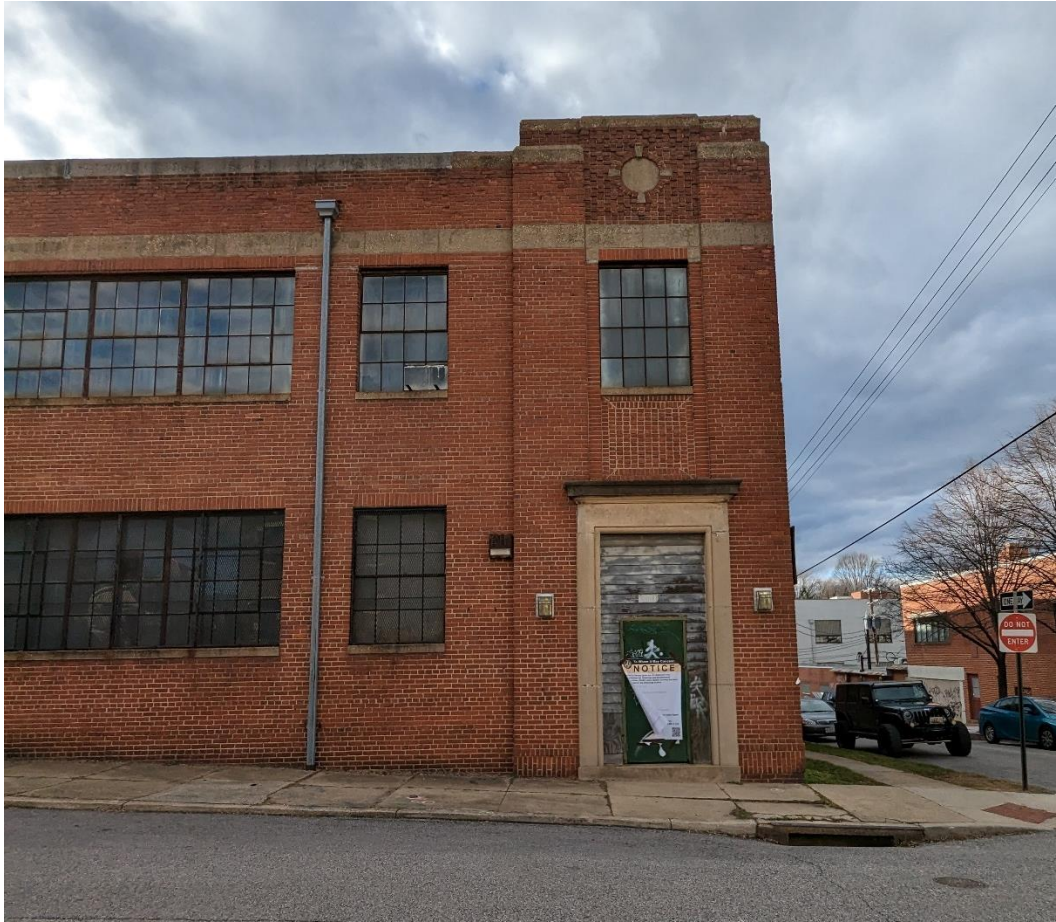
Image 16: Main entrance to the building on Elm Street.
