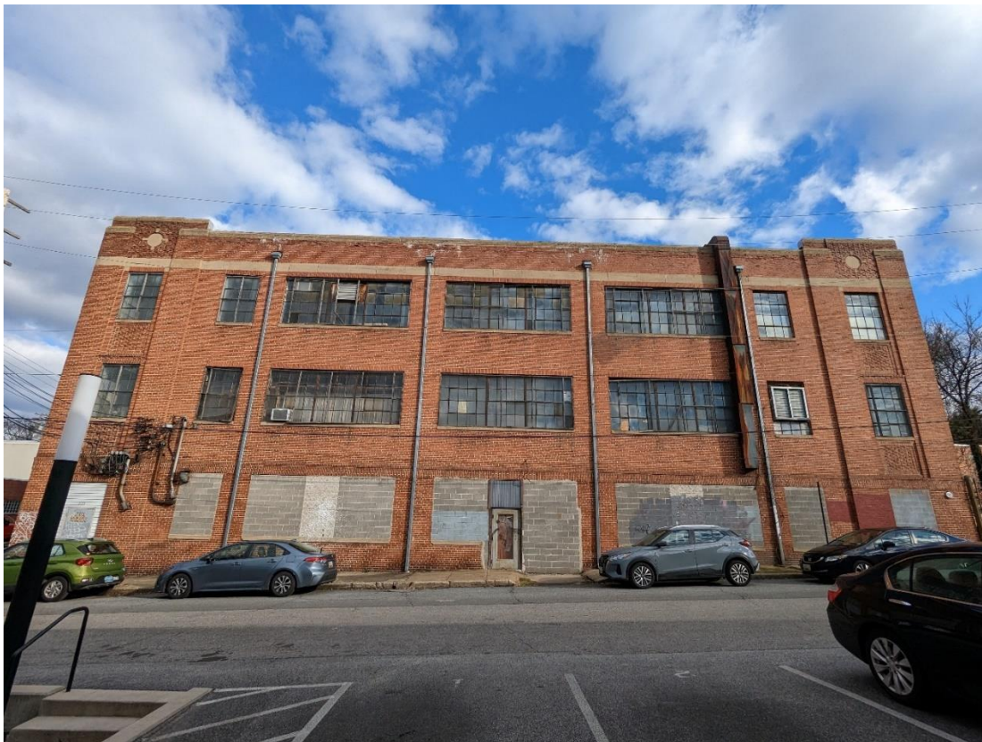
Image 24: West elevation, facing Falls Cliff Road.
