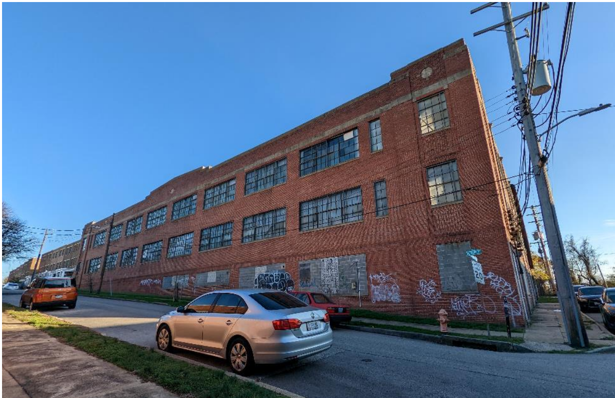
Image 20: North elevation, facing 32 nd Street.
